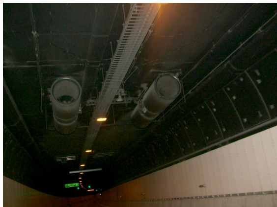
Figure 1, Brisbane's Clem 7 tunnel
